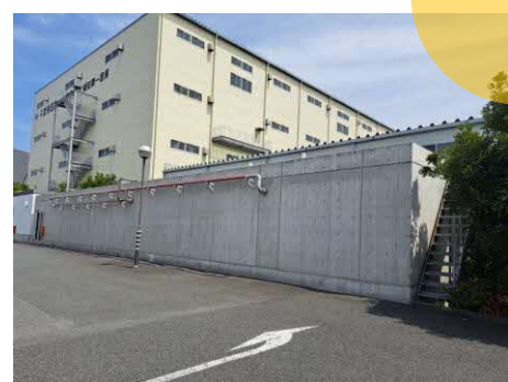
厨房除害設備
